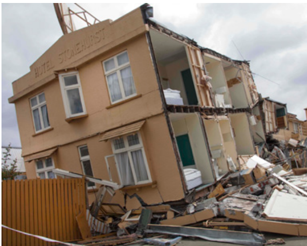
Damage in Christchurch from the February earthquake.
