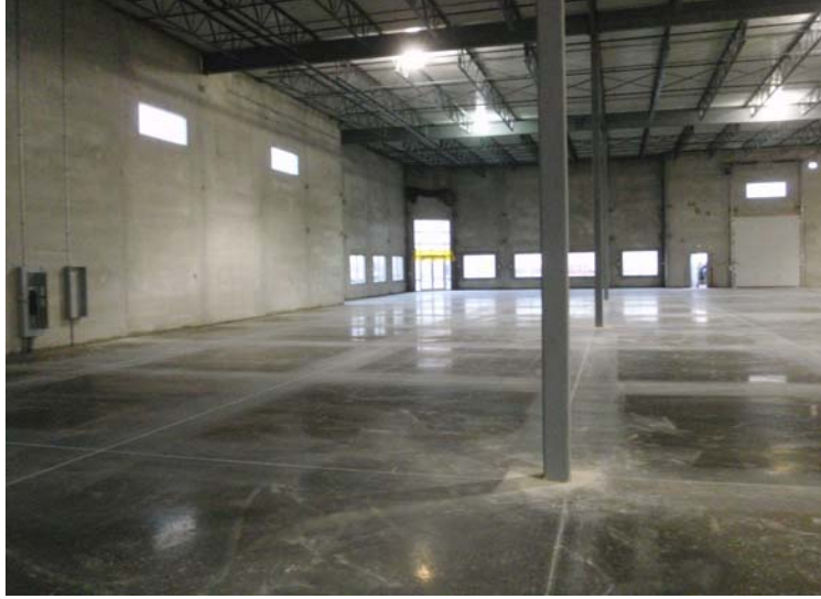
Small 14' x 13' sawcut panels
