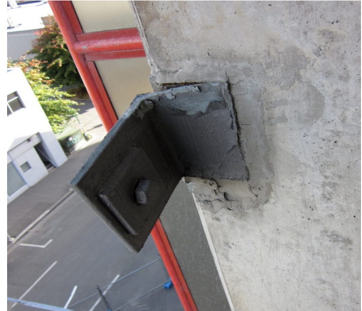
Deformed connections
