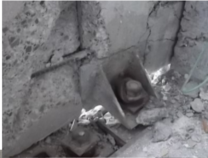
Cracked and spalled concrete
