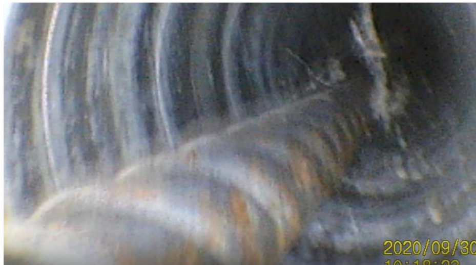
Figure 4: Example photograph of a starter bar within a Drossbach duct without any grout present
