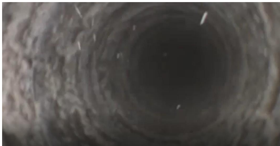
Figure 6: Photograph of an ungrouted duct with no starter bar present within
