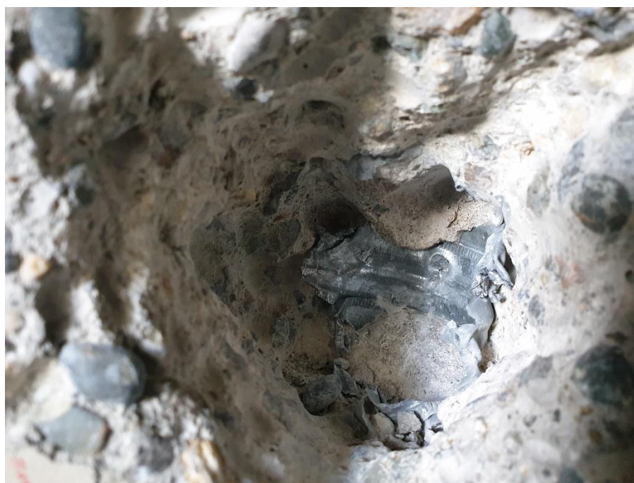
Figure 7: Photograph of a grout filled duct that has been broken out and found to have no starter bar within the duct
