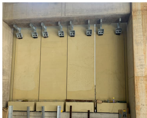
Typical Façade connections during installation
