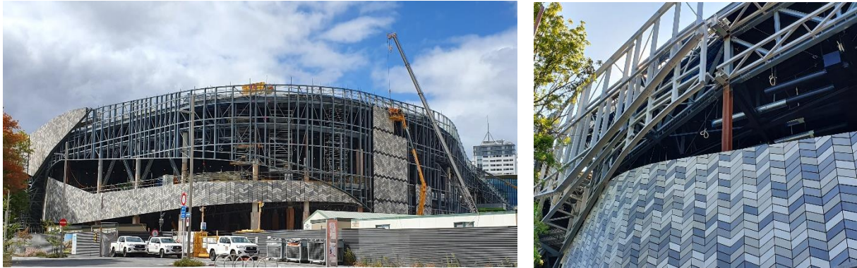
Figure 11: Erection of multi-layered façade ribbons
