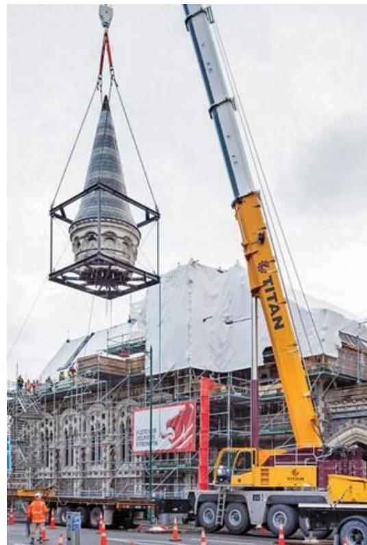
Figure 2: Reinstating the Clock Tower spire during restoration construction
