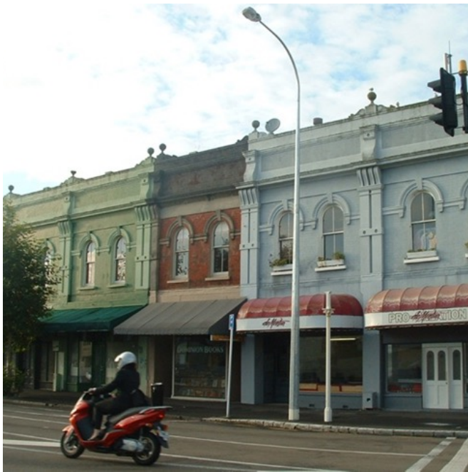
Figure 1: Typical low-rise URM buildings
