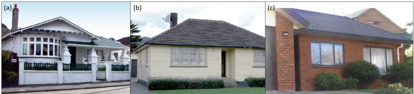
Figure 1: Predominant residential housing typologies: (a) typical 1930s timber frame bungalow; (b) 1940-1960 timber frame house; (c) post-1980s brick veneer timber frame house [7].
