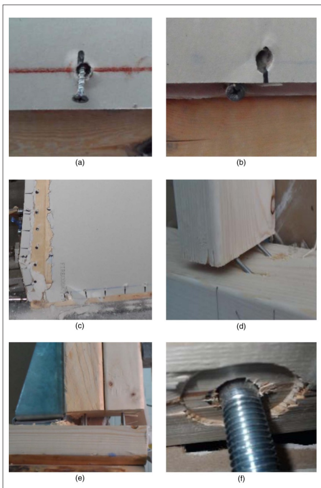
Figure 15: Typical plasterboard sheathed shear wall (overseas cases) failure modes: (a) fastener bending; (b) panel edge tear out; (c) plasterboard fissure failure; (d) end nails yielding and withdrawal; (e) hold-down deflection; (f) wood crushed by anchor bolt [15].
